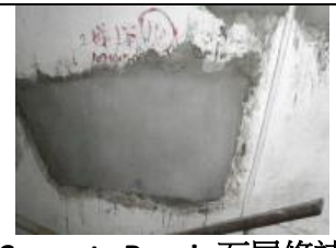
Concrete Repair 石屎修補
