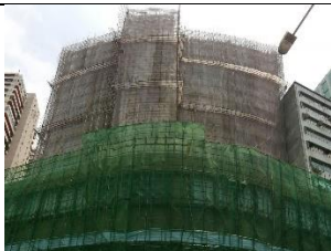
Scaffolding 外牆棚架
